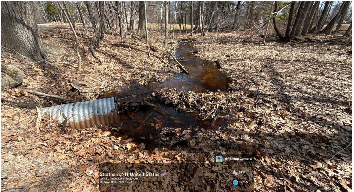
Photo #1: Looking north at proposed Wetland Impact “A” for culvert upgrade.
