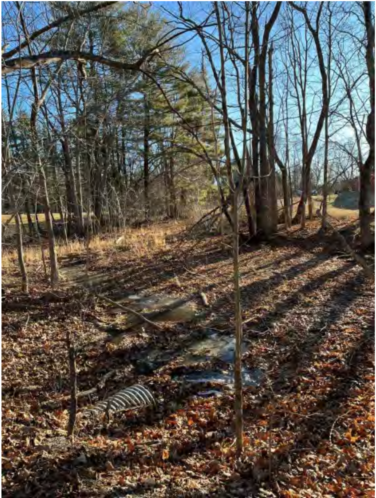
Photo #2: Looking east at same wetland (Wetland Impact A).
